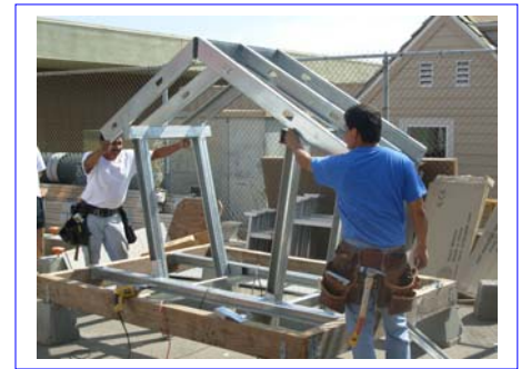
Landscape / Auto Cover is checked for square by Nicholas Lane Contractors
