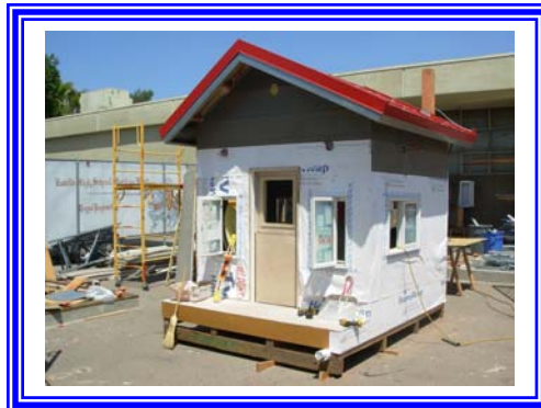
Oracal Quality Finish installs the Dutch Door
