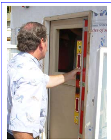
Oracal Quality Finish checks the door installation
