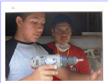
BITA student installs Dutch Door hinge
